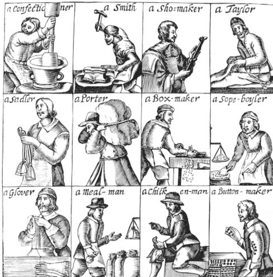
Visual Connection Archive
